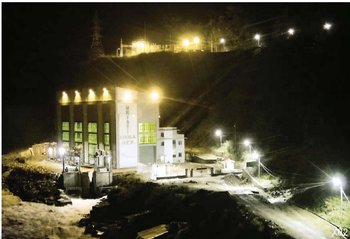
MISTRI KHOLA HEP POWERHOUSE & SWITCHYARD
