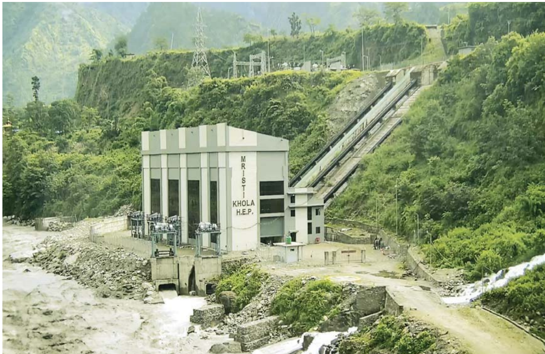
MISTRI KHOLA HEP POWERHOUSE & SWITCHYARD
