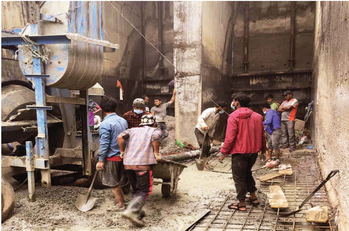
UNDERSLUICE REPAIR WORKS AT TADI KHOLA HEP
