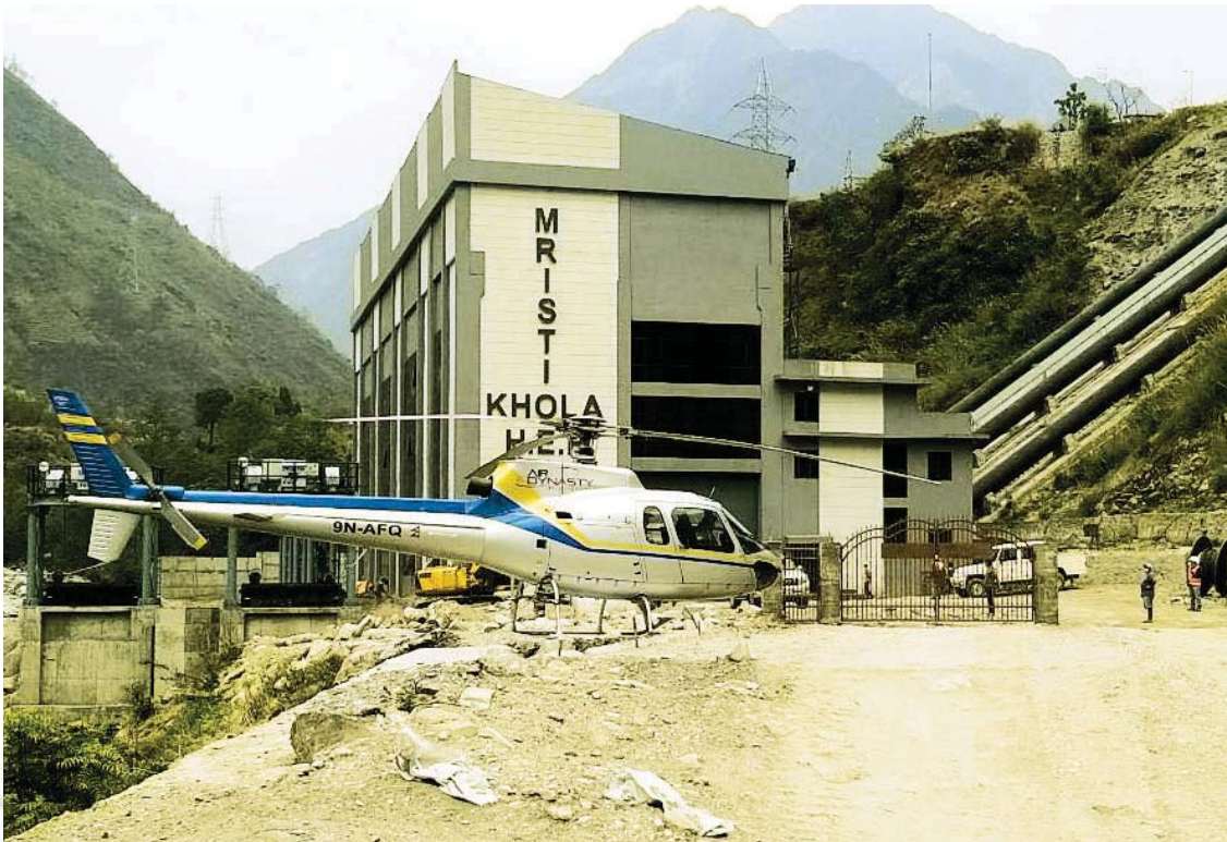
HELIPAD IN POWERHOUSE AREA
