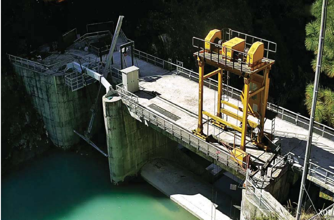
MISTRI KHOLA HEP DAM & INTAKE
