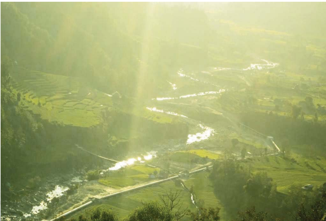
TADI PENSTOCK ALIGNMENT
