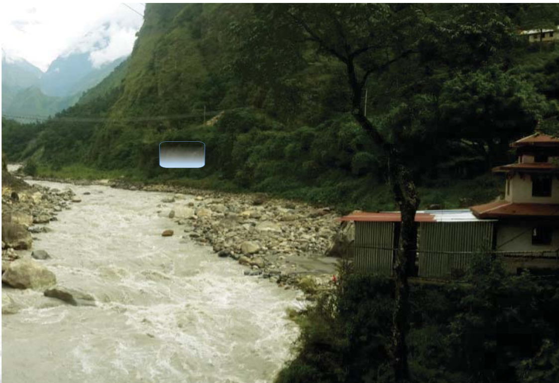
POWERHOUSE AREA OF MISTRI KHOLA-2
